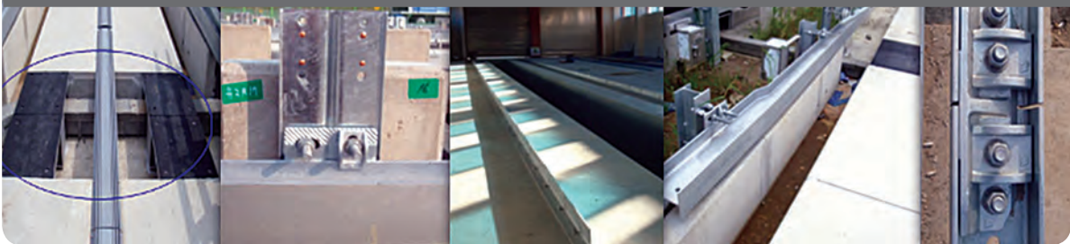
Driving lane color Guide rail mounting plate Inspection area guide rail Approach guide rail Joint plate
