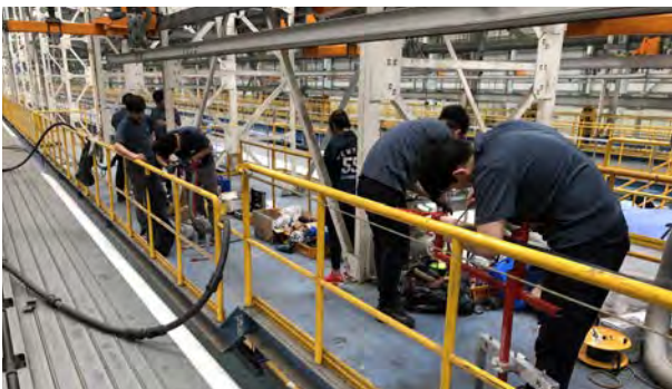
Step 3: On-site execution: Assembly and approval of prototype. Electrical routine test of new installed components on the train. Training of local maintenance personnel. On-site execution of the complete retrofit by ALPHA-ET engineers or by trained local maintenance personnel.
