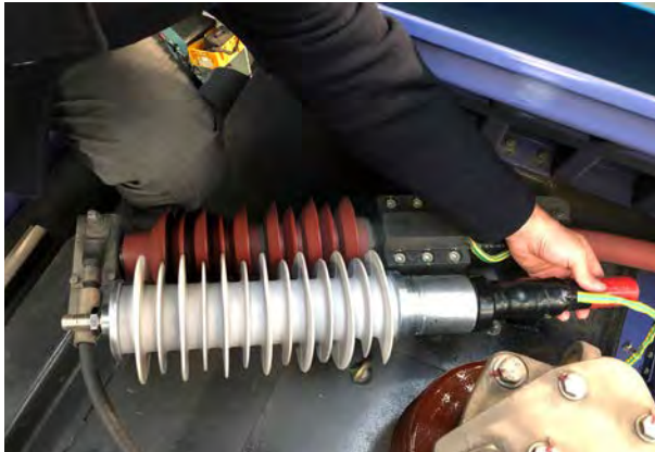
Step 1: Analysis of the installed components, on site on the train or at ALPHA. Examination of the interchangeability of components.
